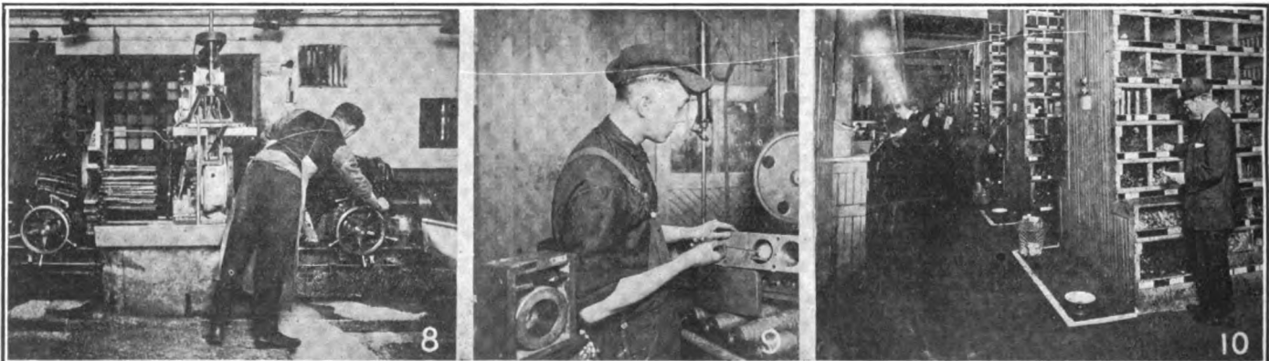
Key to illustrations: 8, Working with multiple drills on a clutch housing; 9, Inspection of twin-six cylinder after boring, with gauge checking to a thousandth of an inch; 10, Stockkeeping where there are thousands of bins numbered and contents catalogued
